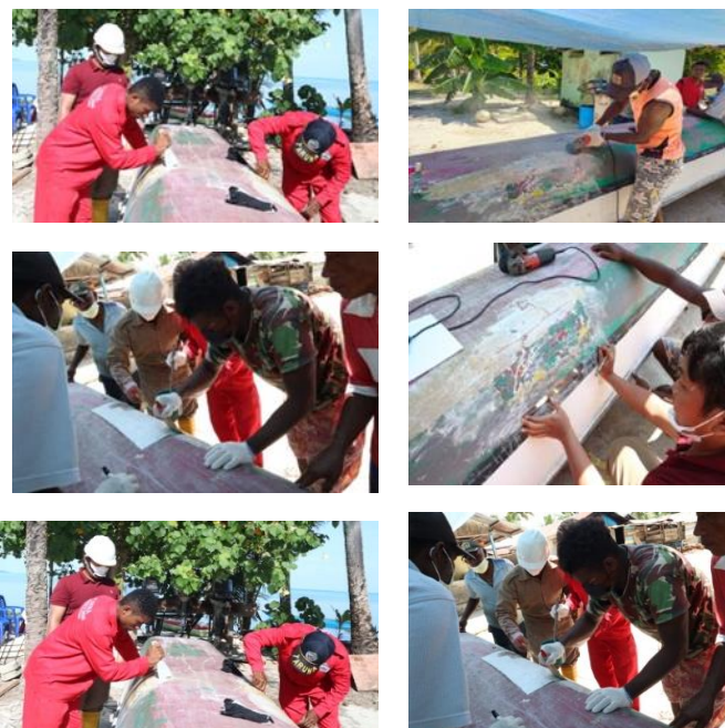
Gambar 7. Proses perawatan kapal fiberglass
