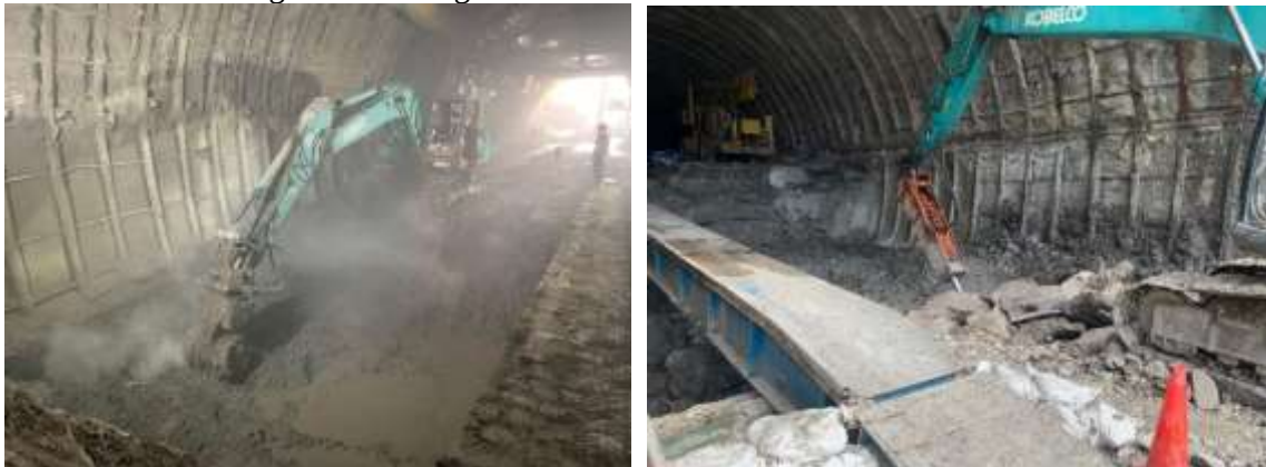
Gambar 10. Galian Invert/Lower Tunnel
