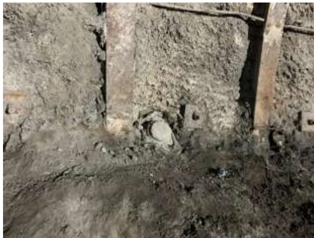
Gambar 9. Grouting Angkur
