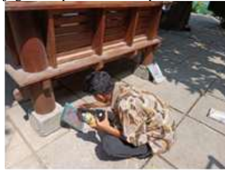
Gambar 7. Proses pewarnaan dan finishing coating.
