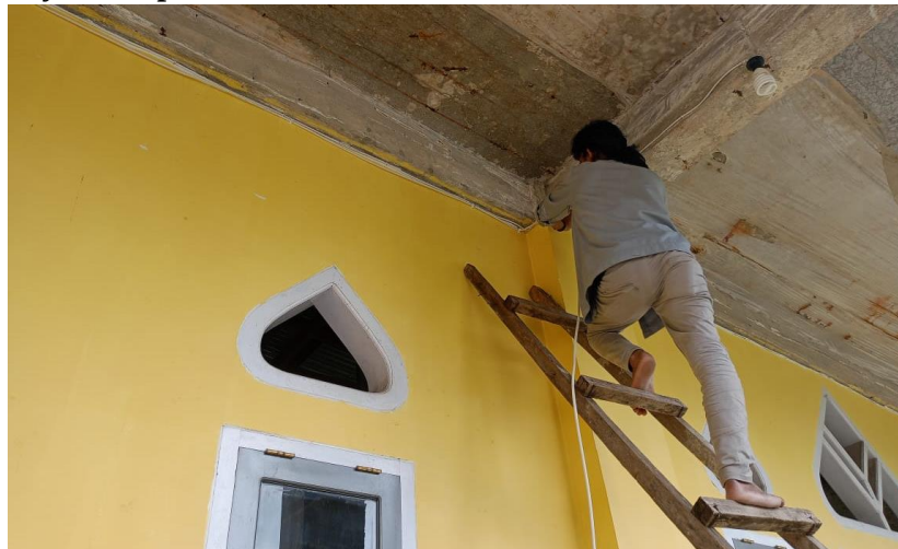
Gambar 7 Pemasangan Instalasi emergency backup system
