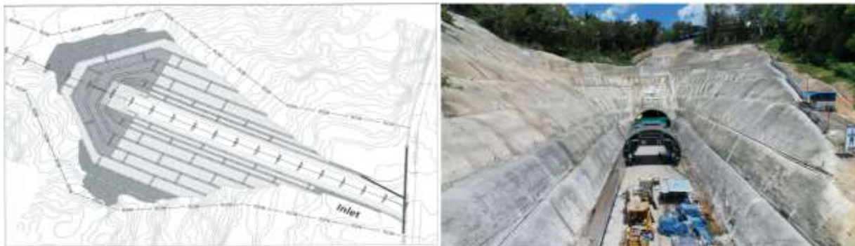
Gambar 4. Plan Shotcrete Inlet
