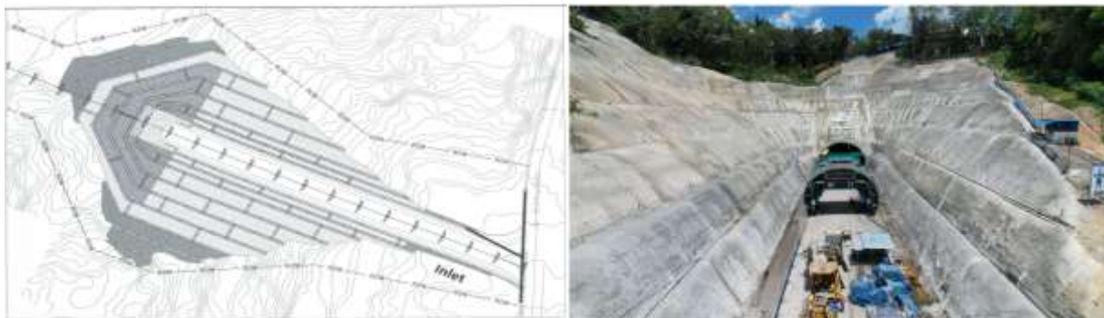
Gambar 4. Plan Shotcrete Inlet
